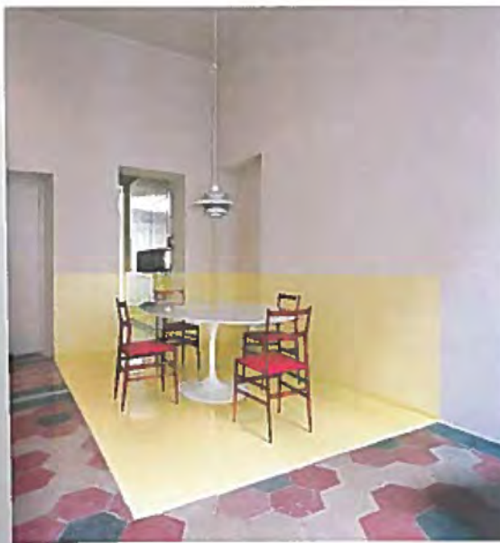
maat architettura, Apartment, Turin, Italy, 2006. Epoxy resin coating on floor and wall, satin finish, color code: SIKKENS G8.30.85 (4041 color concept)
